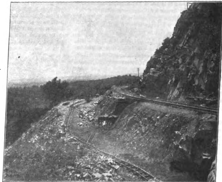
FIG. 9.—ROCK EXCAVATION AND FILL AT DEVIL'S NOSE View showing temporary openings under the track to reach the excavation on the inside of the curve.
