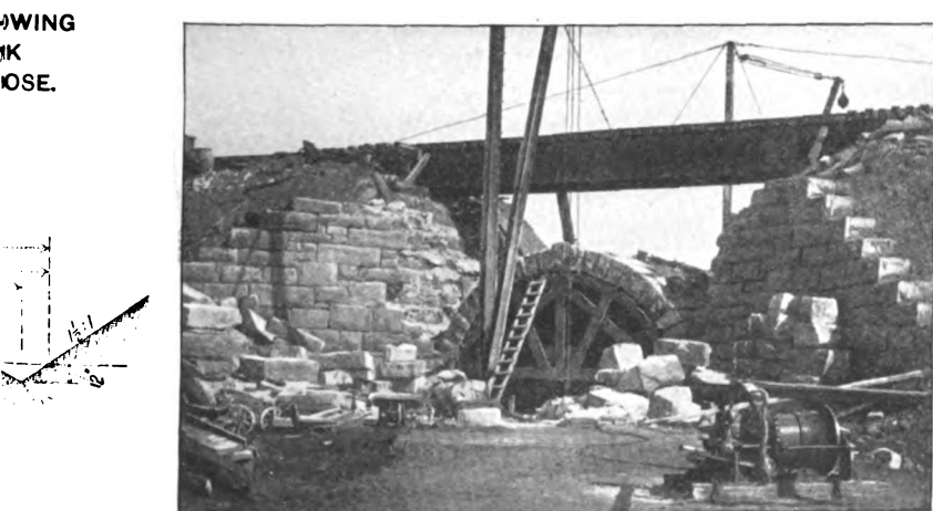
FIG. 12. VIEW SHOWING MANNER OF CARRYING THE TRAFFIC WHILE REBUILDING A 24-FT. ARCH CULVERT.
